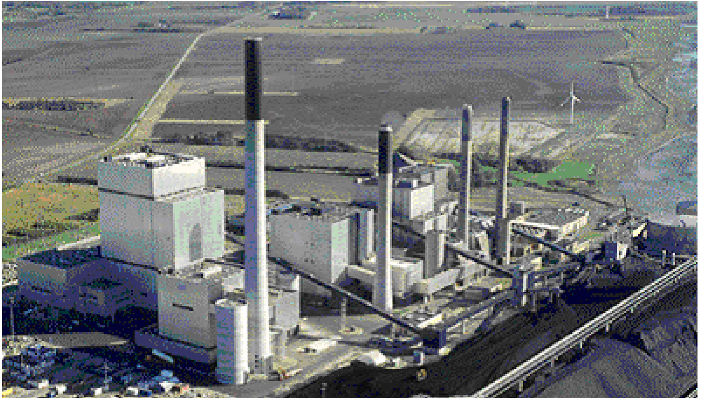
Figure 2: AD 700 ultra-supercritical coal fired power plant
